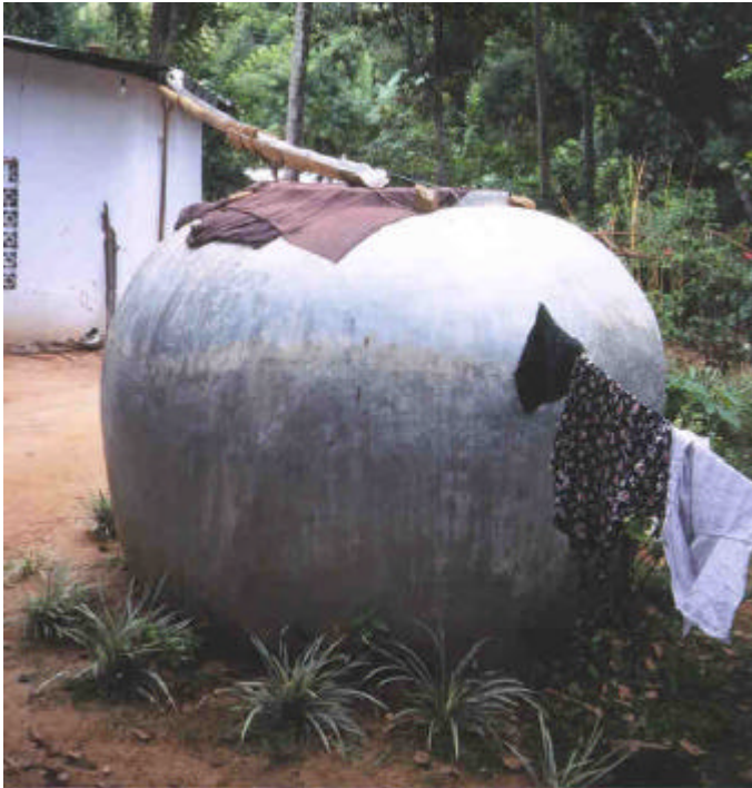
Figure 15: A finished Pumpkin tank
