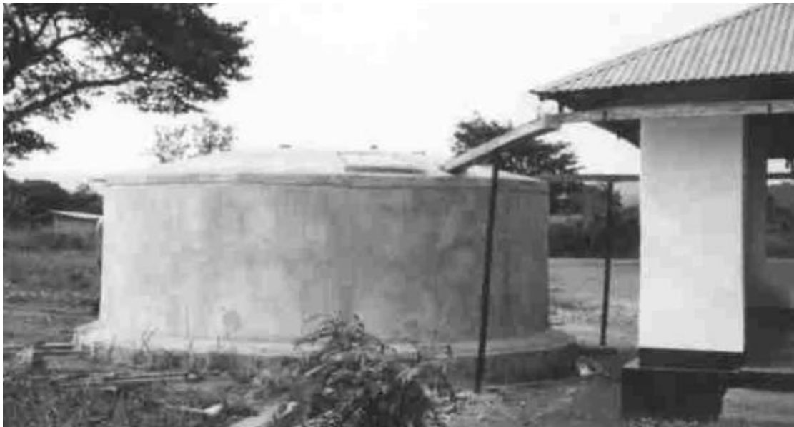
Figure 12: Ferrocement tank in Ruganzu Village
