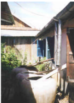
Figure 13: small jars used in Cambodia as part of a multi-sourced water supply
