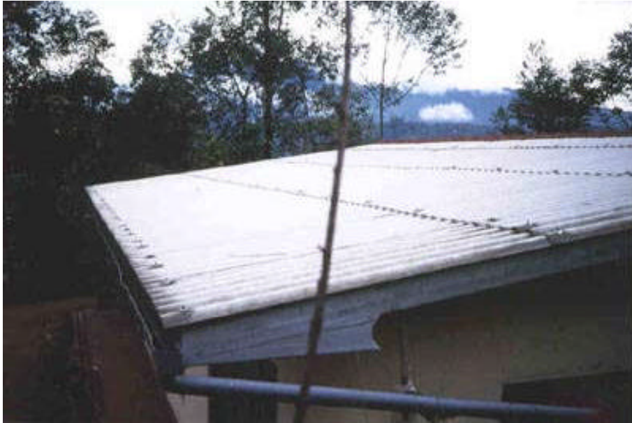
Figure 4: A typical corrugated iron sheet roof showing guttering
