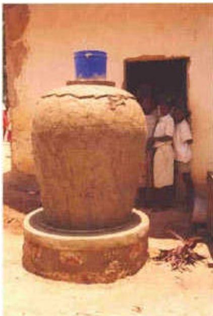
Figure 18 – 'Thai Jar' being built as part of a Water and Sanitation Programme in Tanzania
