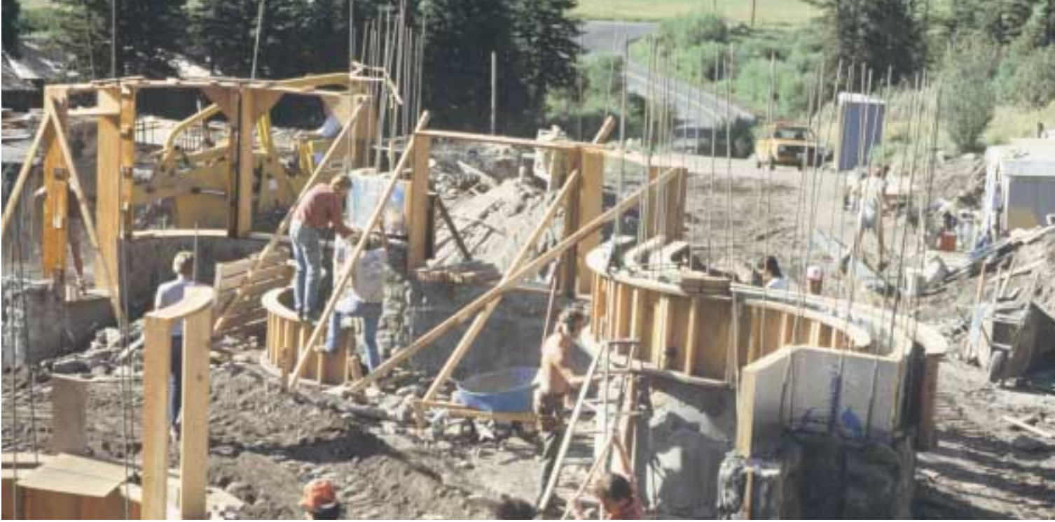
RMI headquarters under construction, summer 1982.
