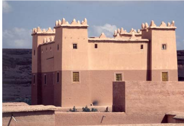
Figure 1: House with stabilised soil render in Atlas Mountains, Morocco. Photo credit: CRATerre/EAG
