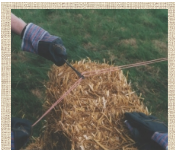
baling needle: this home-made tool allows you to cut and re-bind bales to any size necessary to fit a gap or a corner.
