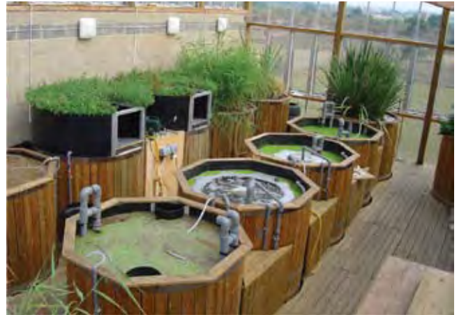
Photo 8 Green Water Treatment Plant, credit: David Triggs
