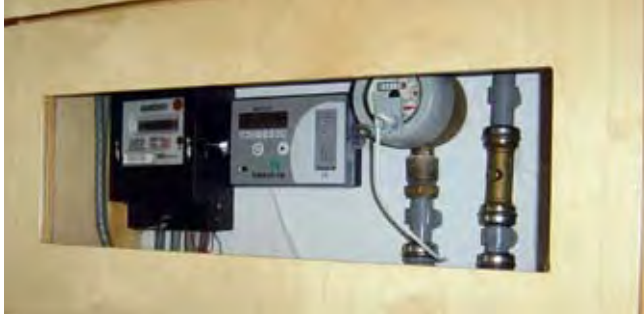
Photo 5 Meters in BedZED house, credit: Christian Lewis Searle
